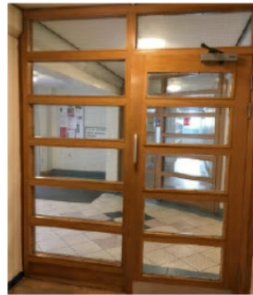
2 - View into entrance lobby
