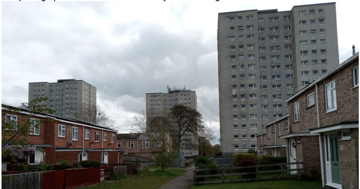
Site photograph 06/05/2021 from the west looking east
